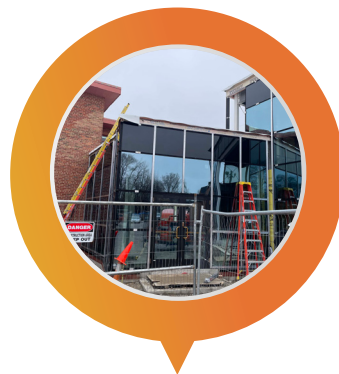
Pause in Construction 2020
